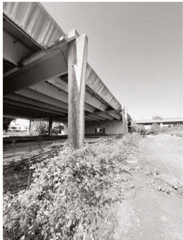
3 – PILASTRO-ALBERO GIGANTE INCASTRATO AL PIEDE, RASTREMATO SUPERIORMENTE PER L'APPOGGIO DELLE TRAVI PRINCIPALI PRECOMPRESSE A "Y" ROVESCIATA
